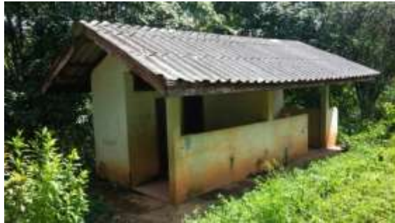
The old toilet building
