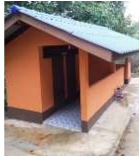
Renovated toilet building
